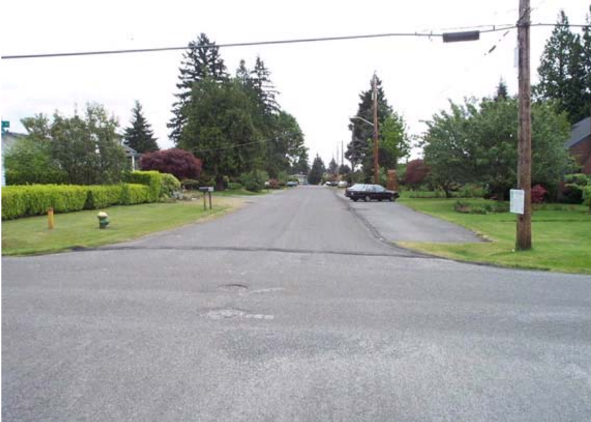
Figure 4. SEA Streets Project, Seattle Washington. A typical residential street, pre-LID application.
