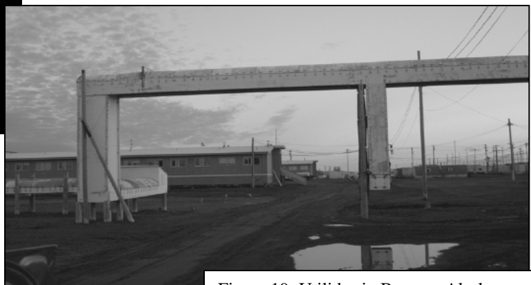
Figure 19: Utilidor in Barrow, Alaska
